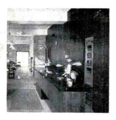
COMPLETE SOUND SYSTEM recessed in one cabinet in the wall behind the reception counter of the Trenholm Motor Lodge. Note bank of four individually-controlled AM-FM radio receivers. At the left of the counter is a paging microphone.
