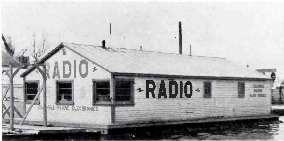
THE FLOATING SHOP of Columbia Marine Electronics with drive-in facilities for customers. There is a 38-foot well inside to permit working under cover. Other boats can tie up alongside.
