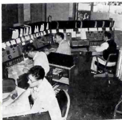
NERVE CENTER of the communications department of Santa Clara County.
