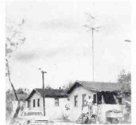
HELIX ANTENNA on roof of home at Furnace Creek Ranch in Death Valley, California, 178 feet below sea level, said to provide reliable reception from Los Angeles stations 180 air miles away. (Courtesy JFD)
