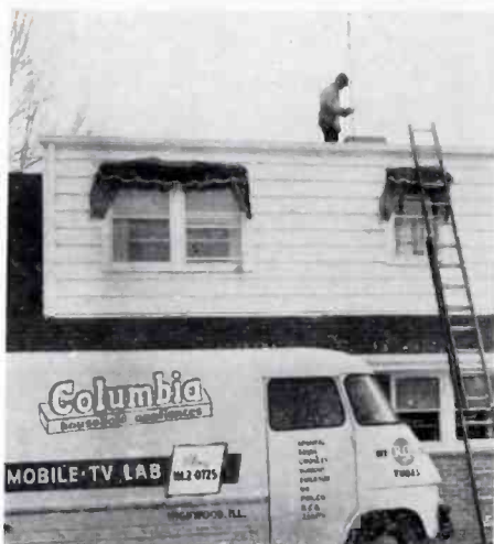
INSTALLING A TV-set coupler on antenna mast.
