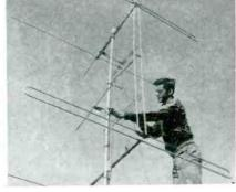
Vertical mast and cross-arms of antenna of *Perma-tube* (electricweld steel tubing coated with a plastic type rust-resisting finish) developed by Jones & Laughlin Steel Corp.
