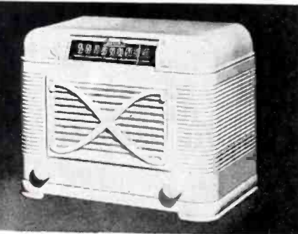
Five-tube farm model battery receiver recently announced by John Meck Industries. Uses 5 miniature tubes that draw 1.4 volts.
