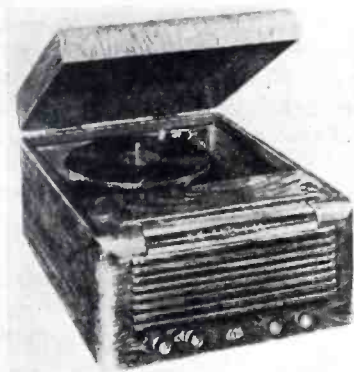
Below, Garod 6A1 a-c/dc super with untuned r-f stage.
