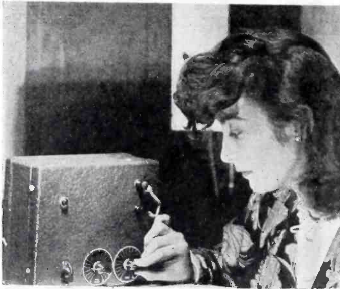
A-C operated multivibrator with adjustable pitch control.
