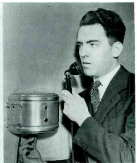
Fig. 6. Bart Heaney, dispatcher, makes a remote emergency announcement at one of the twenty-two microphone stations in the terminal.
