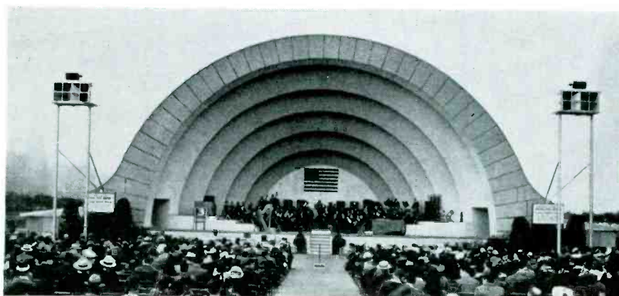
Fig. 9. Chicago's Grant Park employs several amplifier systems to reinforce musical offerings of guest conductors and soloists. Separate speakers are used for low and high frequencies.
