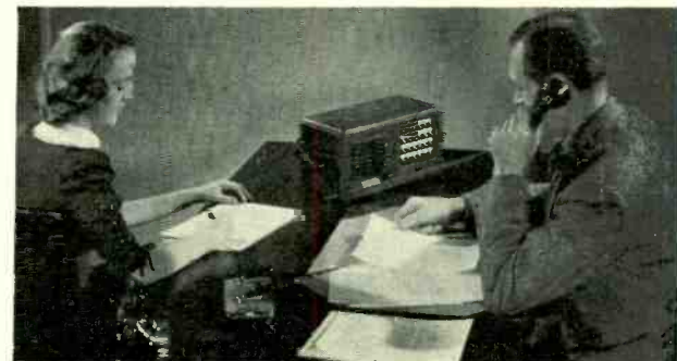
Fig. 17. Signal lights, annunciator drops, elimination of manual push-to-talk switch operation, and privacy through use of a hand-set when desired, mark the latest intercom equipment.
