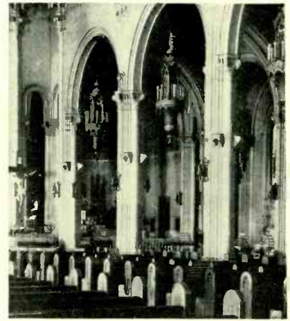
Fig. 20. The interior design of St. Peter and Paul's Cathedral, San Francisco, Calif., presented a difficult acoustic problem which was overcome by a carefully planned RCA sound system. Speakers are mounted in appropriate housings on the pillars.
