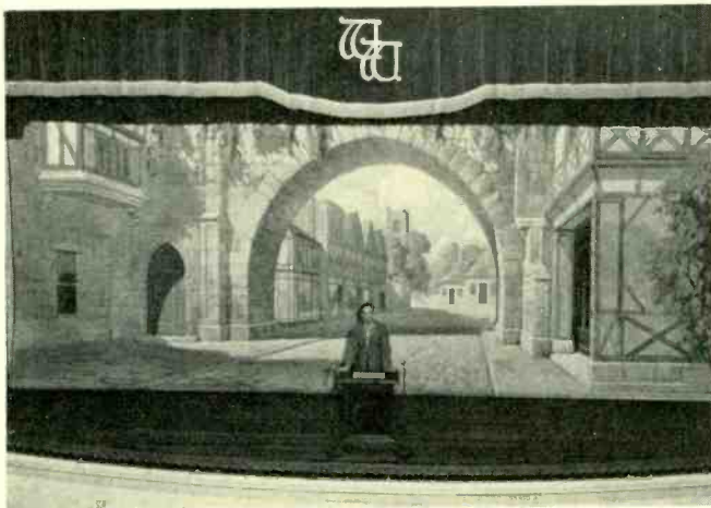
Fig. 22. Uni-directional microphones aid materially in overcoming feedback tendencies inherent in many school auditoriums. They solved the problem for the Radio Equipment Co., Dallas, Texas, in making this installation in the Woodrow Wilson High School. Shure Unipler mikes were used.
