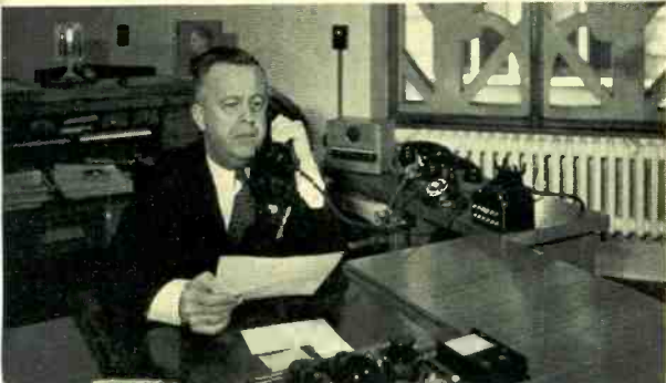
Fig. 16. An unusual intercommunication installation by Morlen Electric Co. in the Metropolitan Life Insurance Co.'s main offices links five executives' desk sets with 10 talk-back speakers in the supply department, the latter so sensitive to pick-up that supply clerks can talk back from any point without interrupting their work.
