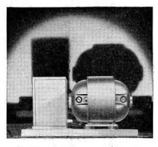
The Carter Genemotor. The double filter is in the case to the left of the motor-generator
