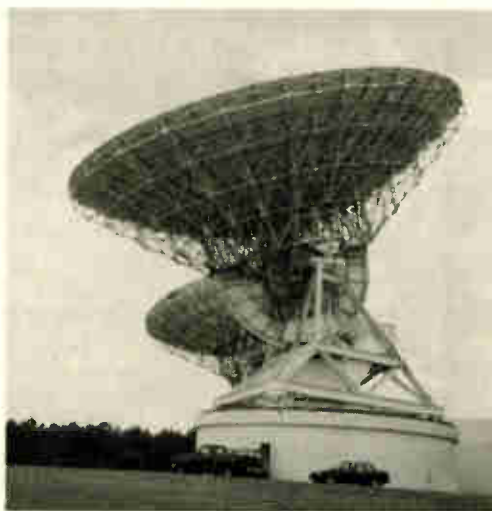
The two 105-foot dishes at Woodbury.
