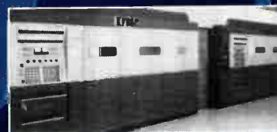
100 kW SW Transmitters
