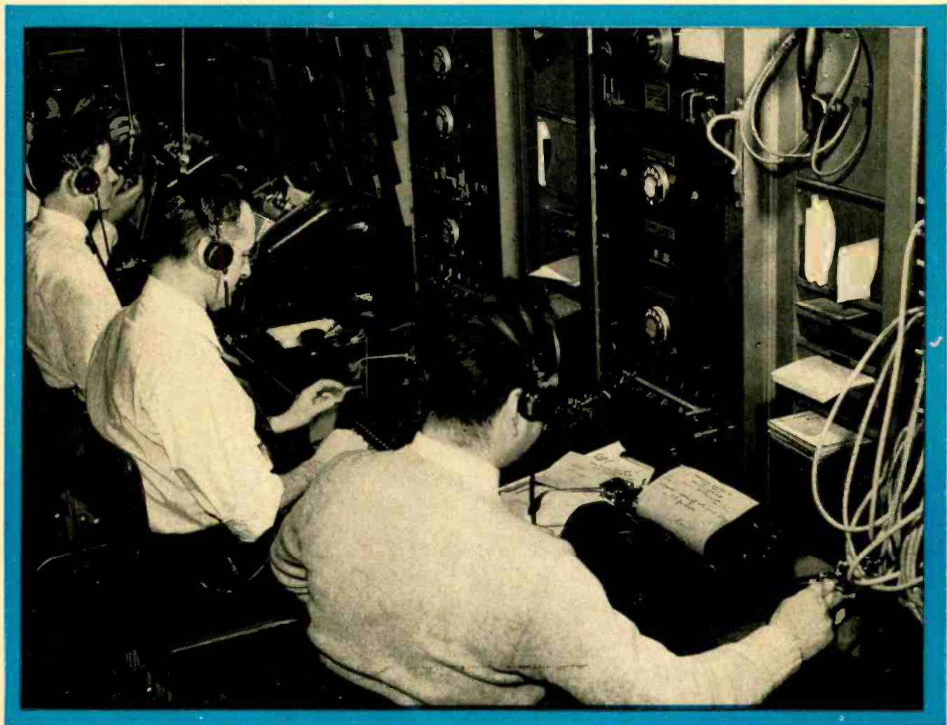
Wilcox Installations. Photo, courtesy American Airlines
