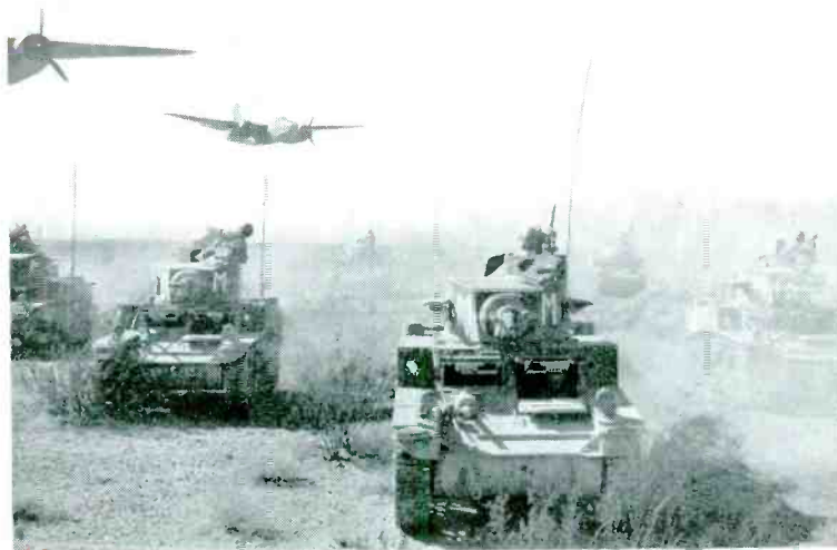
At a desert training center, planes are shown strafing a formation of tanks with their whip antennas depicting the commands being given by radio.
