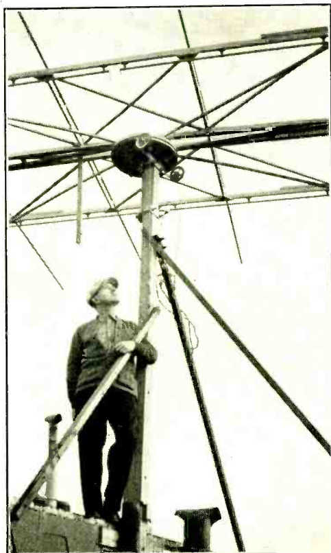
W6FK makes final inspection. Note detail of the rotary head and the method of mounting it on the mast.
