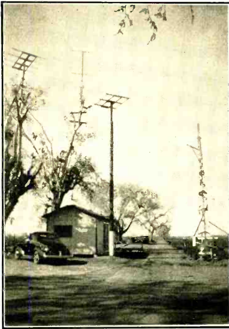
The arrays at W6QLZ, Phoenix, Arizona. Reading from left to right they are: the 56-Mc. 4-element rotary, the 56-Mc. lazy H, and the 28-Mc. 3-element rotary. The rhombic terminates just under the lazy H.
