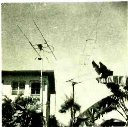
W4DRZ's twenty and ten meter rotaries, and horizontal two-section 8JK for "five."
