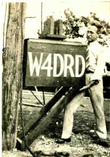
Showing the motor-driven rotating head before being hoisted up the telephone pole which supports the 20-meter installation at W4DRD. An ohmmeter-type direction indicator is part of the control box at the operating position.
