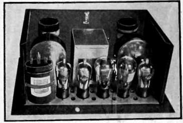
View of the HB Compact AC Model, the tubes being, left to right: 124 first AF, 345 power tube, 280 rectifier and 234 RF. The subpane 9%x14%", ret everything save the speaker is in this small space!
