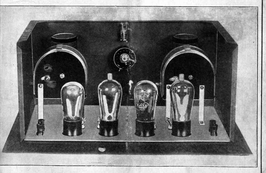
Rear View of Exceptional 4-Tube Set Using Two 222 Tubes, One 240 and One 112A. See pages 3, 4 and 5.
