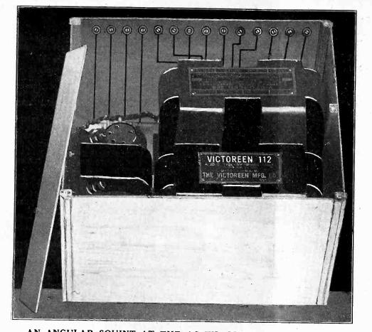
AN ANGULAR SQUINT AT THE AC FILAMENT SUPPLY AND AUDIO AMPLIFIER SHOWS THE TOP AND THE PARTITION OF THE SHIELD REMOVED. PLACEMENT OF THE 112 TWO-STAGE AUDIO AMPLIFIER AS SHOWN KEEPS THE GRID LEADS AWAY FROM THE FILAMENT TRANS-FORMER. THE BINDING POSTS TOWARD THE LEFT ARE FOR FILAMENT SUPPLY OUTPUT, TO SERVE EXTERNAL TUBES. THOSE TO THE RIGHT ARE INPUTS FROM A B POWER DEVICE.
