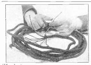
In a battery cable there is considerable capacity between the various conductors. This capacity minimizes the pick-up to which the cable is subject. The pick-up can be still further decreased by grounding one of the conductors in the cable.
