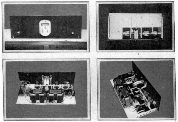
LOCALIZED TUNING OF THE AC SET RESULTS FROM GAUGING TWO OF THE TUNING CONDENSERS AND USE OF THE HAMMARLUND DRUM DIAL (TOP LEFT). THE BASEBOARD IS CUT OUT AS SHOWN (TOP RIGHT) TO PERMIT LEEWAY FOR DRUM AND CONDENSERS. BOTTOM VIEW IS SHOWN. THE FILAMENT TRANSFORMER IS AT RIGHT, THE AUDIO UNIT AT LEFT, IN LOWER LEFT PHOTOGRAPH. AN ANGLE VIEW IS DEPICTED IN LOWER RIGHT.
