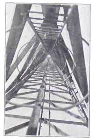
A BIRDSEYE VIEW up one of the 820-foot steel masts of the new radio station at Hillmorton, near Rugby, England. This is the first step of an imperial chain of radio transmitting stations, which will send commercial radio messages around the world. The complete station covers an area of over 900 acres. The power output of the station is 100 kilowatts. The signals are transmitted on a wavelength of 6,000 meters. (Acme.)
