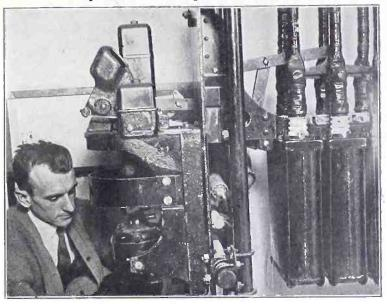
ONE of the motor-operated oil switches of WJZ's super-power station is at left. Although in a separate building, this, like all other switches, is operated from the control board in the operator's room. Note the huge condensers at right. (Kadel & Herbert.)
