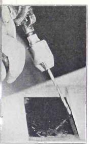
HE PHOTOGRAPH shows how to II a hole in a panel, without having o drill slip oll over the panel, thereby atching it and delaying the work. In a place of wood snug up against place where the hole is to be illed. Tighten down with a vice. In you can drill the hole without y fear of the drill slipping, as it will rest up against the board.
