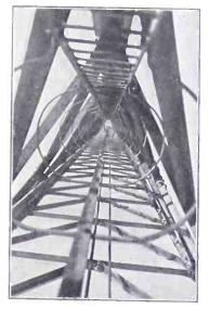
A BIRDSEYE VIEW up one of the 820-foot steel masts of the new radio station at Hillmorton, near Rugby, England. This is the first step of an imperial chain of radio transmitting stations, which will send commercial radio messages around the world. The complete station covers an area of over 900 acres. The power output of the station is 100 kilowatts. The signals are transmitted on a wavelength of 6,000 meters. (Acree.)
