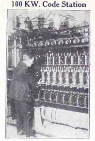
A GENERAL view of the power unit in the new and world's most powerful commercial wire!ess station, at: Hillmorton, England, near Rugby. The station opened on New Year's day. The wavelength is 6,000 meters, power 100 kw. (International Newsreel)
