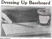
PUTTY may be used as a filler to plug up a hole in a wooden baseboard.
