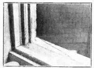
HERE is an actual photograph of aerial leadin. Notice the broken wire. The fabric of the covering keeps the line mechanically intact, but the broken elec-trical lead makes the set in operative. A leadin strip or tube should have been used, thus preventing the wire from rub-bing against the stone sill.
