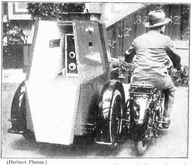
A SHIELDED transmitter and receiver in a sidecar is the latest radio novelty in Germany.
