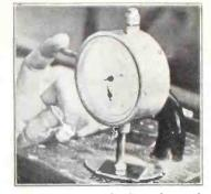
WHEN a mica fixed condenser is carefully made the thickness of the mica is measured with a meter and voltage is applied for electrical test. (International Newsreel)
