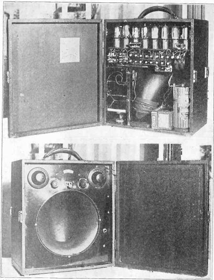
A COMPLETE 8-tube Super-Heterodyne compactly arranged in a 16x18" valise. The top picture shows the inside rear view of the receiver, the eight 199 tubes being supported on a piece of hard rubber panel. The lower photo shows the front panel, with speaker built in. The two dials control variable condensers.
