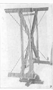
FIG. 6-Side view of loop, showing winding method.
