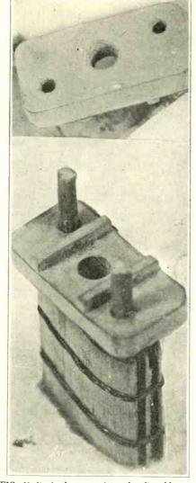
FIG. 11 (top) shows a piece of soft rubber, cut to fit the outside container. Details of the con-tainer are shown in subsequent photos. Fig. 12, lower, shows a close-up of the completed elements.
