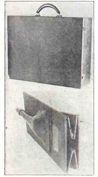
THE CARRYING CASE (above) makes a neat "package." Below is the folding horn, which fits inside the case.
