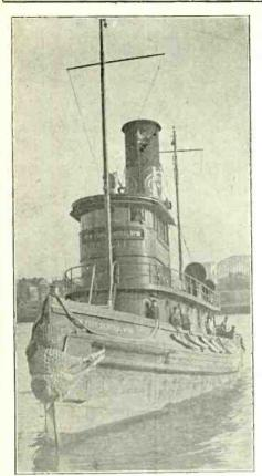
THE PROUD TUGBOAT, first to be equipped with radio for commercial purposes in New York Harbor, is known as New York Central No. 18. Orders directing the movement of the tug are re-ceived on a short-wave set, instead of being tels-phoned over land wires and the message "called for" at a pier. (Kadel & Herbert)
