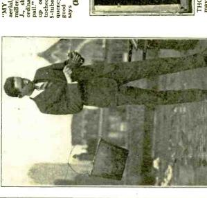
"MY idea of a good aerial," said Harold Heltmiller, of Jersey City, N. J., shown at left, "is an ordinary empty iron water pail." So he rigged one up on the roof and attached the lead-in to his 5-tube tuned radio-frequency set, using also a good ground, Now he says he wouldrit change.
