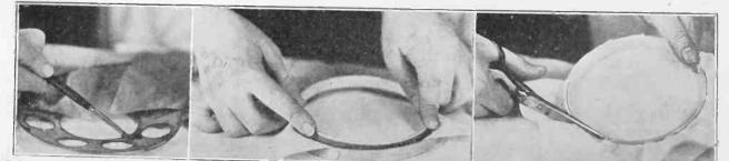
FIG. 5, left, shows how, after the flaps are glued together to restore the card hoard disc to as a firm unit, the shellac is applied. Fig. 6, center, shows the method of using the embroidery hoops to enclose the speaker diaphragm, which is parchment, gold gauze, Georgette crepe, China ailk or other silk. Bond paper may be used. The excess is cut away. (Fig. 7.).
