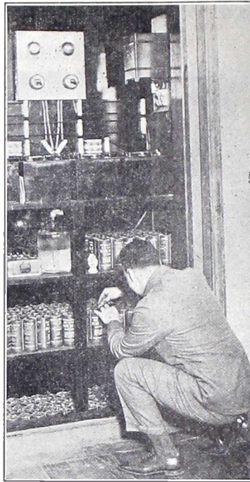
THIS GREAT array of dry cell supplies power for a Super-Heterodyne, employing peanut tubes and a powerful 4-stage amplifier in the Cornell Club in N. Y. City. Note the large number of 1½-volt dry cells. (Kadel & Herbert)
