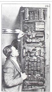
TURNING a dial or two to tune in a station is easy enough, but much that is complicated must go into a broadcasting station to render your personal ease possible. W. E. Novy is exposing the back of WRNY's main control panel. This station, operated at the Hotel Roose-velt, New York City, by "Radio News," through the enterprise of Hugo Gerns-back, editor, is one of the most compact in the world.
