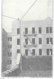
FIG. 5, showing a view of one of the poles. The guy wires are difficult to see, due to the similar background. Note the height of the pole, and how the antenna is continued right through the insulator.
