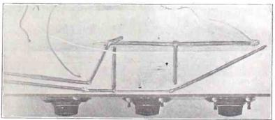
FIG. 5, an excellent view of the bottom of the set. Note the filament leads, identified by the heavy black leads. For the filament wiring use No. 14 insulated wire. Also need by the neary black leads. For the niament wiring use ivo. 14 insulated wire. Also note the leads coming through the holes in the baseboard, which are connected to the various batteries. DO NOT FORGET TO PUT TAGS ON THE LEADS, so that you won't blow out your tubes.
