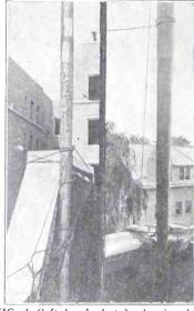
FIG. 1 (left hand photo), showing how one of the poles is held in place. This is at the slanting portion of the roof. Note the large amount of rope holding the pole. Fig. 2 (at right), showing how the poles which is at the cornice of the roof, looks. Note the guy wire coming down from the pole. The slot which is below the wire wrapped around the pole, was purposely it looks like. Also note the peculiar middle section of the pole.
