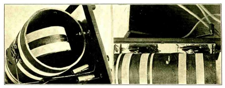
THE ROTORS (Fig. 9, at left) are wound on 2½" diameter tubing, 1¾" high, and have 17 turns each. Notice that pigtail connections are used, as these afford secure contact. The coiled pigtail may be plainly seen at left in Fig. 9. The objects at lower right in this photograph are fixed condensers. The photograph at right (Fig. 10) shows the aluminum shield, placed 1" in front of the tuner unit and connected to ground.
