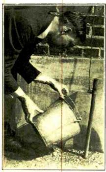
RAYMOND B. WALES, of 911 23rd St., Washington, D. C., shows the world how to make a good outdoor ground. To make sure that the earth surrounding the pipe is always a conductor of electricity, a bucketful solution, commonly called bluestone, and which is cheap, should be poured around the pipe. The solution prevents corrosion and is highly conductive. An iron pipe is used for ground connection.
