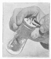
FIG. 2—To prevent circuit noises clean the prongs of the vacuum tube every two months. Good contact in the vacuum tube circuit is very important, if the highest efficiency is to be attained.
