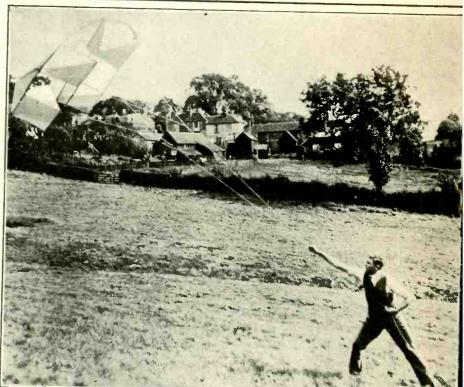
A HUGE KITE was used in recent tests at a radio field day in England for raising a long aerial to a position amid the clouds. A mobile station used the aerial for broadcasting. Note the insulator, at right, on the ground, showing where the aerial wire is joined as part of the kite string, and in this fashion raised. (International Newsreel);
