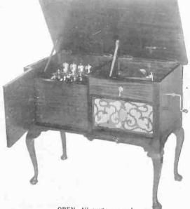
C ABINET 39 inches long, 21 1/2 inches deep, 34 1/2 inches high, fully conceals receiving set, "A" and "B" batteries, also doing away with unsightly horn.
