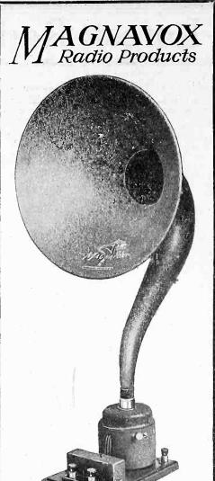
'HE Magnavox Reproducer I illustrated above is the most popular and largest selling Radio Reproducer. R3 has the famous electro-dynamic construction which insures re-creation of programs according to the original pitch, quality and volume.
