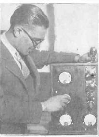
THIS MACHINE, used by Saul Weltzer, New York City dealer, tests tubes for voltage and amperage.
