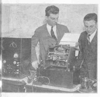
In a recent test in New York City of the invention of William G. H. Finch writer operated at the sending station, two miles away, caused the receiving same words at the same speed—65 a minute. The receiver is called a radio asmitted, instead of by wire, as is now done, on a 60-meter wavelength.
