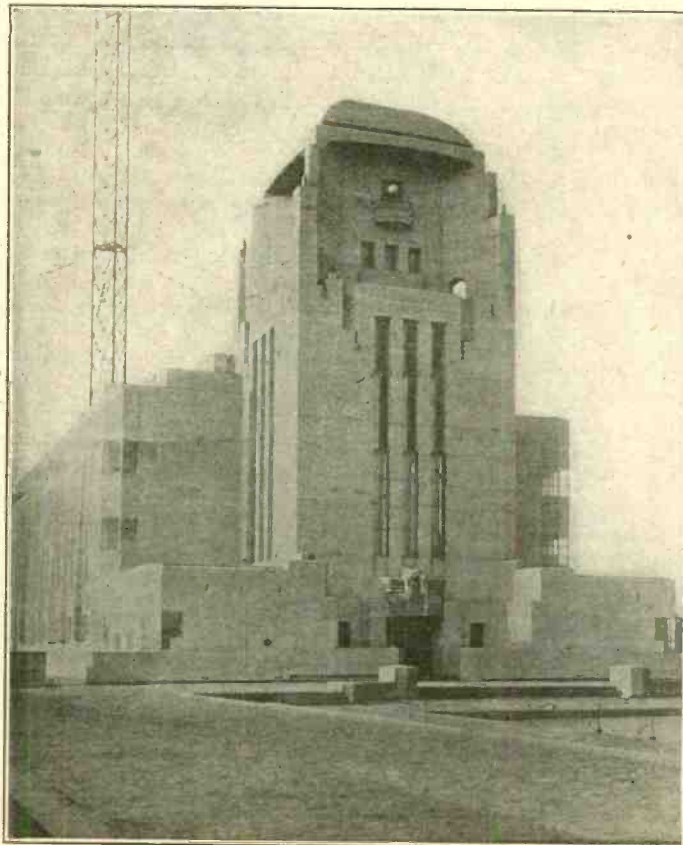
The unique and interesting government radio station just completed at Kootwijk, Holland.
