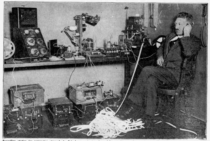
Recording station for comparing atmospheric disturbances at several receiving stations at the same time. The disturbances are charted on a moving strip of paper, as shown, and then compared. Definite time settings are made and the readings can be taken almost simultaneously. The receiver is a typical German experimental station with the addition of a high power audio-frequency amplifier used to furnish current to operate the sensitive recording relay.
