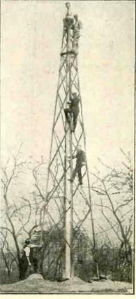
Located in a place which because of its surroundings did not permit the proper erection of an antenna, these members of the Radio Association of Greater New York built this 100-foot mast to get the best results out of their sets. The chief operator of the club, R. May, is seated atop the tower.
