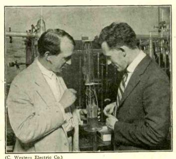
Fig. 3. W. G. Housekeeper (left) and Dr. W. Wilson (right), of Bell System Laboratories, examining the filament—grid assembly of a 100,000 watt water-cooled tube. Mr. Housekeeper is pointing to a copper disc seal which he developed.
