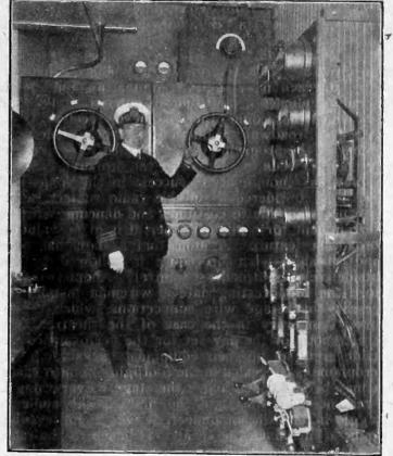
(C. Kadio Corporation of America) High power tube transmitter on the S. S. "Leviathan." The picture shows the chief radio officer, E. N. Pickerill, changing wave length.
