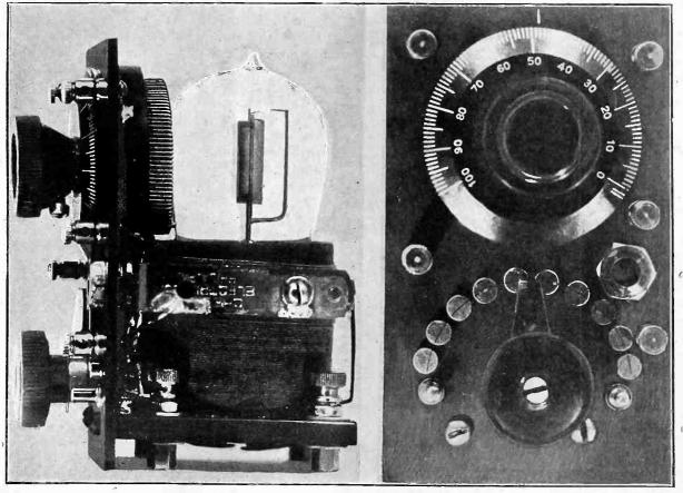
Two views of the portable midget set constructed and described by Dick Roberts. The illustration on the right is a full size photograph of the complete set, and that on the left is a side view of the receiver showing all the apparatus mounted on the base of the socket.
