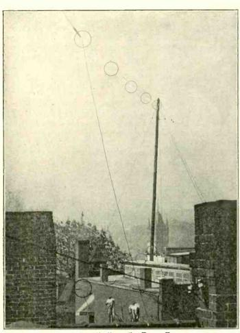
Antenna equipment of WNAV, Knoxville, Tenn. Two cage antennae are used, one as counterpoise and one as antenna.
