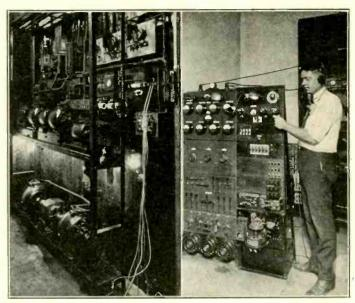
Operating room of station on left, showing generator and controls on back of board. On right is shown the operator listening in on a program by means of plugging in on the power amplifier circuit.
