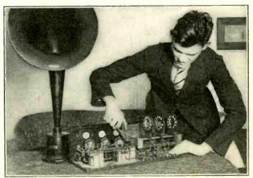
M. Michaels, of New York City, and the "DX Devil" that he has just finished. It is a three-tube circuit, using detector and two stages of audiofrequency, with "Curkoid" inductances. Instead of using them as straight primary, secondary and tickler, he uses the outside as the primary, then connects it variometerwise to the secondary, and leaves the tickler pretty loosely coupled. It is claimed that by so doing, WOC, WOAM and several others can be brought in through local interference.
