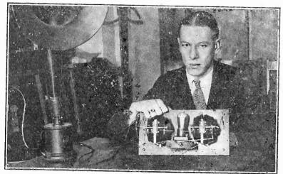
(C. Foto Topics) M. L. Muhleman, the designer of the new one-tube "autoplex" circuit and the completed receiver that he is using as a standard model in designing improvements. The circuit uses neither grid condensers nor grid leaks, making use of only a rheostat, tube, two variometers and one high in-ductance honeycomb coil. The picture shows the rear of set and the location of the apparatus on panel. Simple, isn't it?
